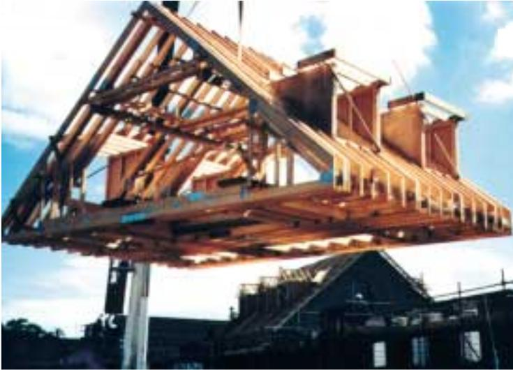
*Above left: An example of ground level erection of “RiR” trussed rafters.*
