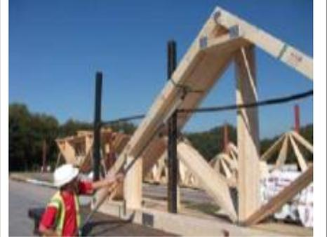
7. The driver will then separate each truss at the heel by separating the individual trusses to the edge of the lorry.
