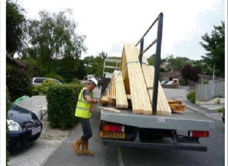
4. DWB will supply truss packs secured to the trailer with blue 3 core rope. You shall familiarise yourself with which rope attaches which pack to the centre bars.
