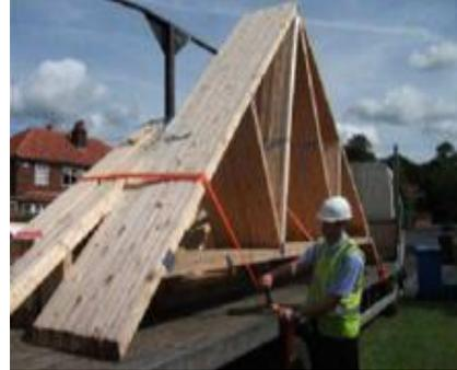
6. The driver will release the blue 3 core rope securing the truss pack to allow separation of the individual trusses.
