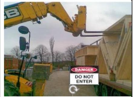
7. The driver will release the individual rope attaching the pack to the bars. This must be carried out from a safe position.
