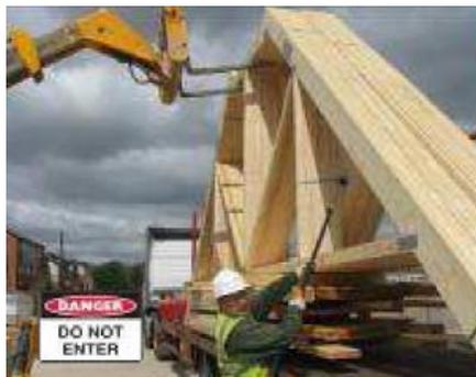
8. The forklift truck operator must lift the trusses from the trailer and then move the trusses to a safe and / or off-load area.
