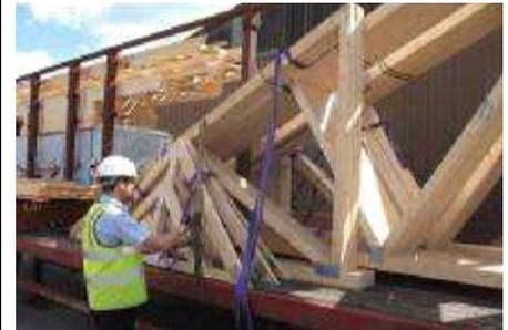
7. The driver will release the individual rope attaching the pack to the bars. This must be carried out from a safe position.
