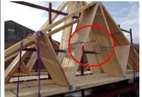
4. Once the order of unloading is agreed between the slinger and driver, the slinger will attach his lifting slings to the crane hooks.
