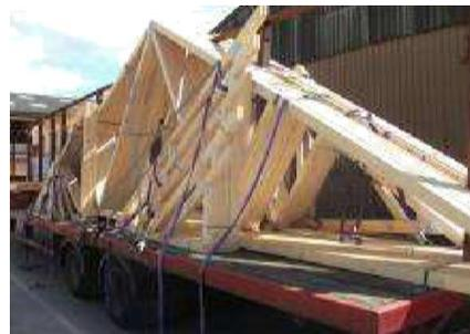
3. DWB will supply truss packs secured to the trailer with 3 core rope or appropriate banding. You shall familiarise yourself with which rope attaches which pack to the centre bars.
