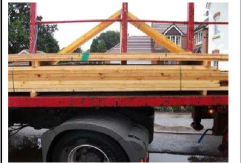
4. On instruction from the site responsible person, the driver will release the transport straps on the side being unloaded ensuring no one is within the danger area as shown in the pictures.
