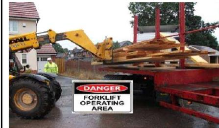
6. NEVER stand between the forklift and the vehicle, do not allow others to enter this danger area. NEVER stand on or under the forks. Ensure the danger area remains clear at all times.
