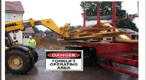
7. The forklift truck operator shall remove the pack into a safe designated area on suitable bearers.
