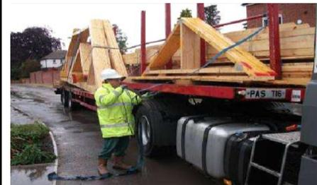
5. The forklift truck operator can now remove the packs and any palletised material from the vehicle. Ensure no one is within the danger area.
