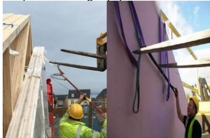
5. The lifting equipment will then take up the slack of the lift, and under instruction from the site responsible person the driver will release the transport straps on the side being unloaded.
