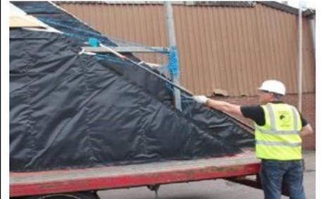
7. The forklift will lift the panel from the bed of the trailer. **NEVER** stand in the danger area where the lifted panel could fall or panels can fall from the trailer.
