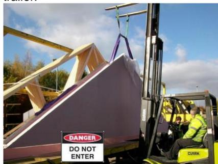
8. Repeat the process for the remainder of the panels. Small clad panels will be secured to a pallet with heavy duty strapping and purple lifting slings attached for ease of off-loading.
