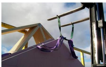
6. On instruction from the site responsible person the driver will release the blue rope which attaches the individual panel to the centre bar, standing outside of the danger area.
