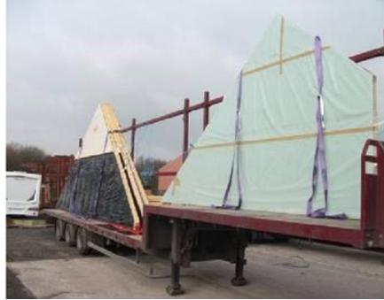
3. The clad panels are individually attached to the centre bar of the trailer with blue rope.
